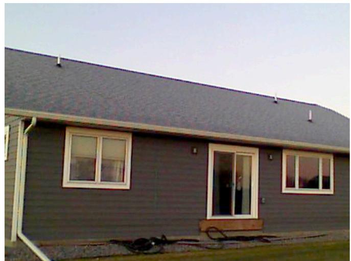
Since SIP roofs provide both the structure and the insulation all in one assembly, there is no need for attics, ceiling insulation, soffit vents, attic vent chutes, ridge vents or attic ventilation. Elimination of these saves construction time, complexity and money. Moreover, not having attic vents keeps insects, rodents and burning fire embers from entering the attic.
