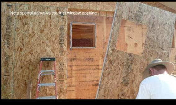
**Figure 8. Window Box with Retrofit Panel**
